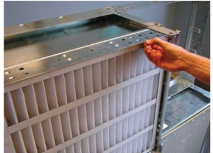
Figure 47: Installation of Prefilter into Frame
