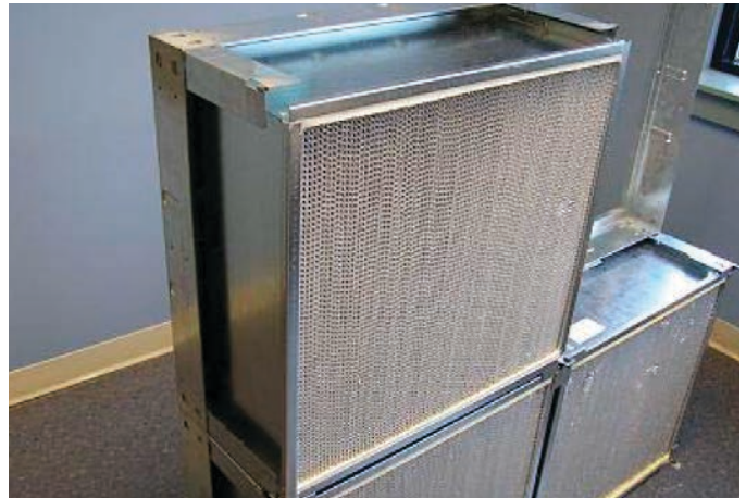
Figure 37: Filter Placed Inside of Frame
