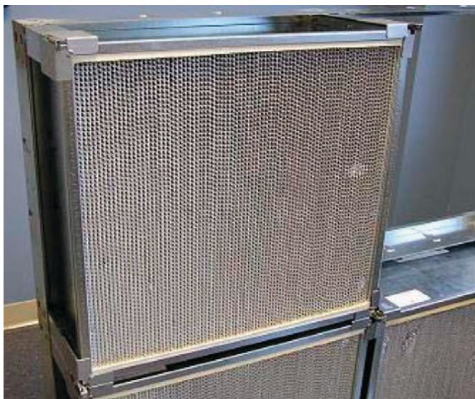
Figure 41: Properly Installed Filter Inside of the Frame
